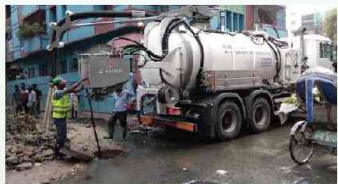
Jet & Sucker Clearing the Drain Blocks
